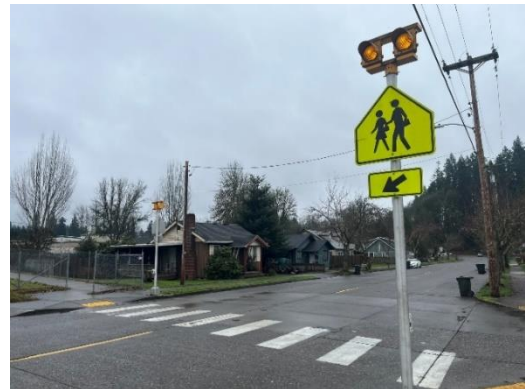
Figure 2: Picture of a flashing beacon; Note that this is not an RRFB.
