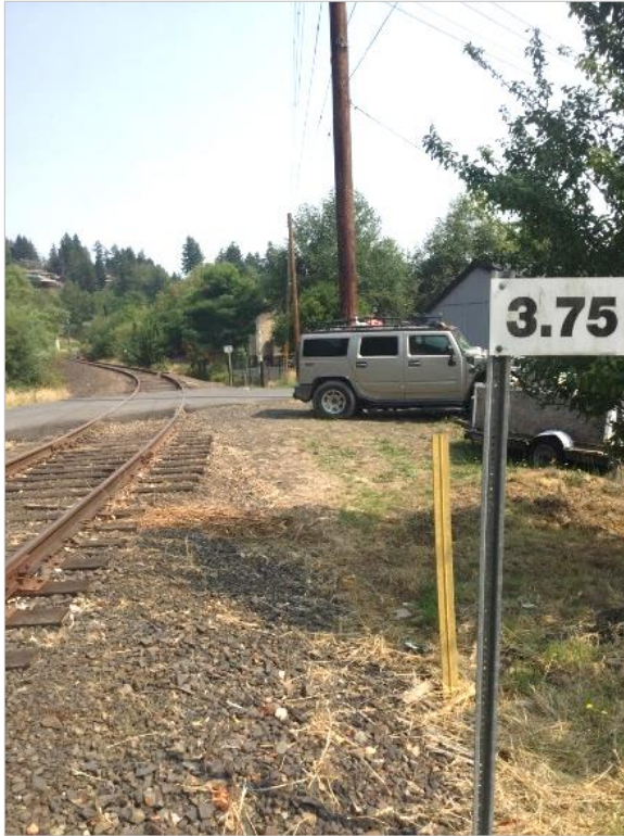
Photo 21. MP 3.75 and Clark Street crossing, looking northeast.
