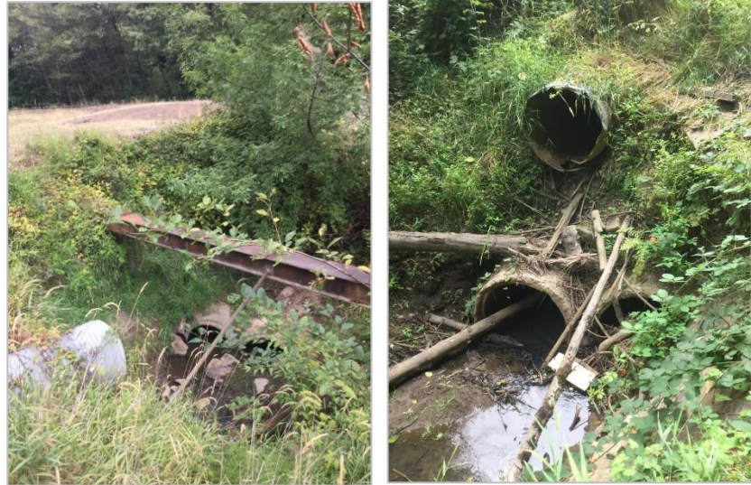
Photo 6. Culverts near MP 4
