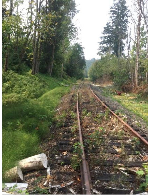
Photo 51. Rail corridor at MP 6.75, with chopped wood in the foreground and fallen trees across the track in the background, looking south.
