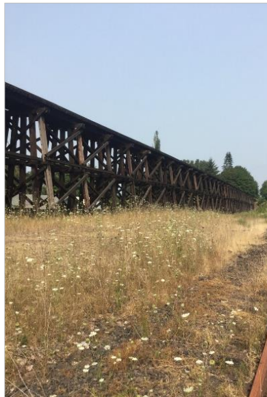
Photo 39. View of wooden trestle, looking northwest.
