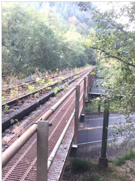
Photo 62. Bridge crossing Ostrander Road, looking south.
