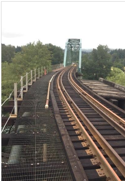
Photo 38. View of rail bridge over Cowlitz River, looking east.
