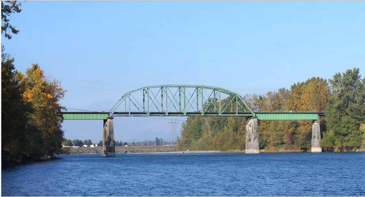
Photo 5. Rail bridge over Cowlitz River, looking north.
