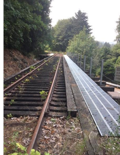
Photo 41. Bridge over N. Pacific Avenue, looking south.
