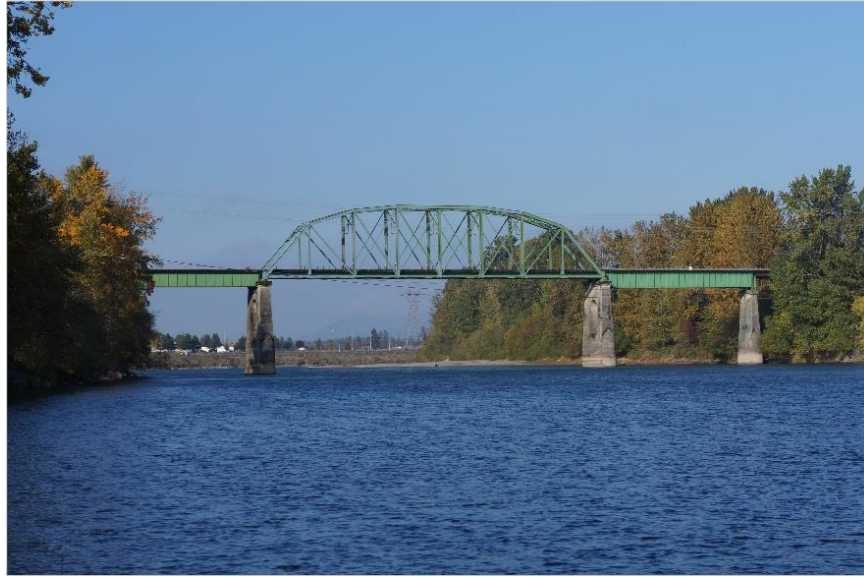
Photo 37. Cowlitz River railroad bridge, looking north.
