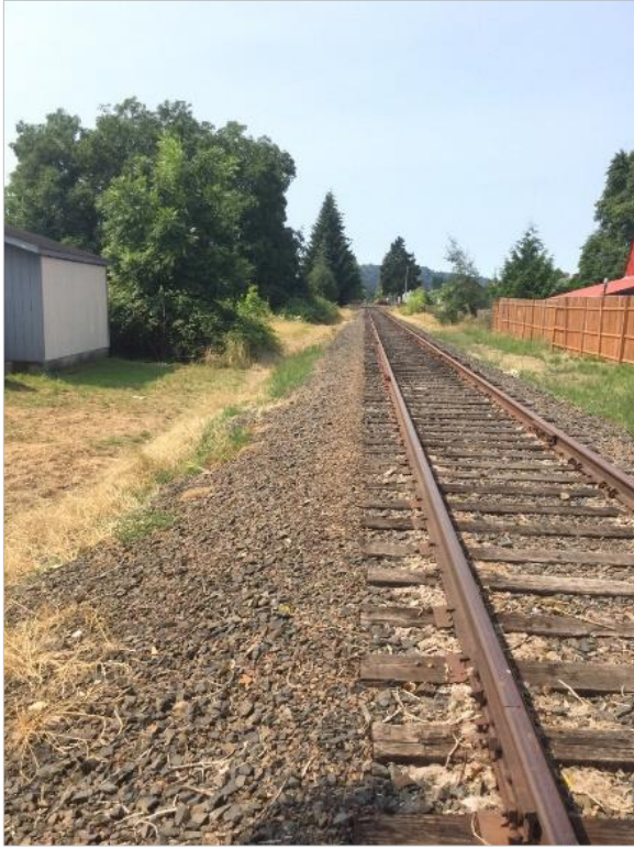
Photo 12. Rail corridor at MP 2.5, looking west.
