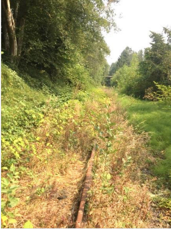
Photo 54. Overgrown stretch of track, looking north.
