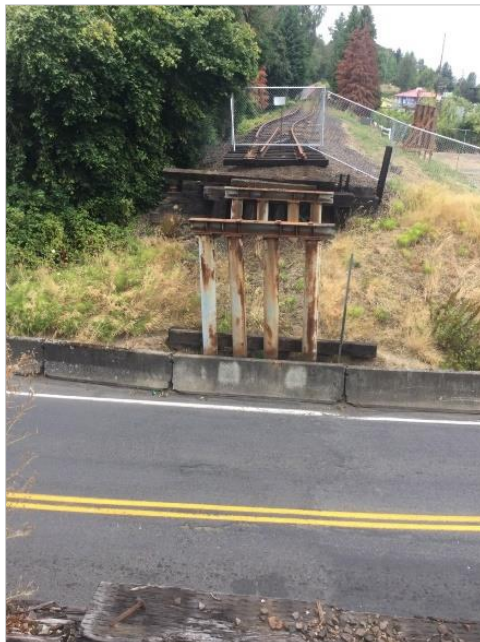
Photo 29. Nevada Drive with no bridge, looking north.
