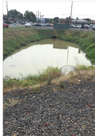
Photo 9. CDID #1 drainage facility and commercial uses, looking southeast.
