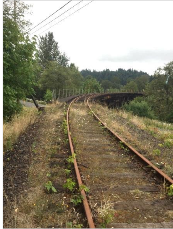
Photo 35. View of trestle over Beacon Hill Road, looking northeast.
