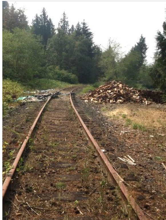
Photo 57. Large woodpile in rail corridor, looking south.
