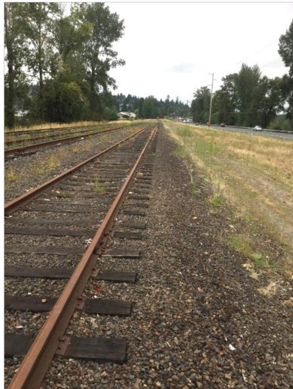
Photo 26. Corridor with three tracks, looking north.
