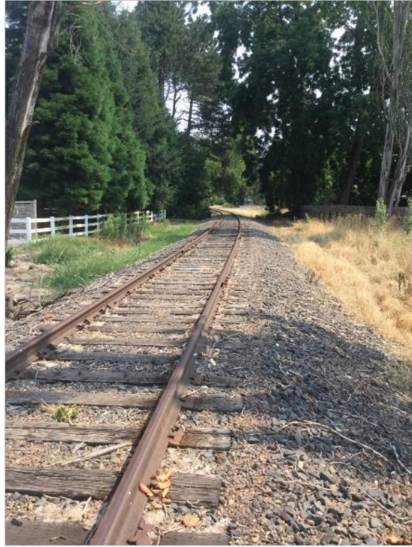
Photo 13. Rail corridor at MP 2.5, looking east.
