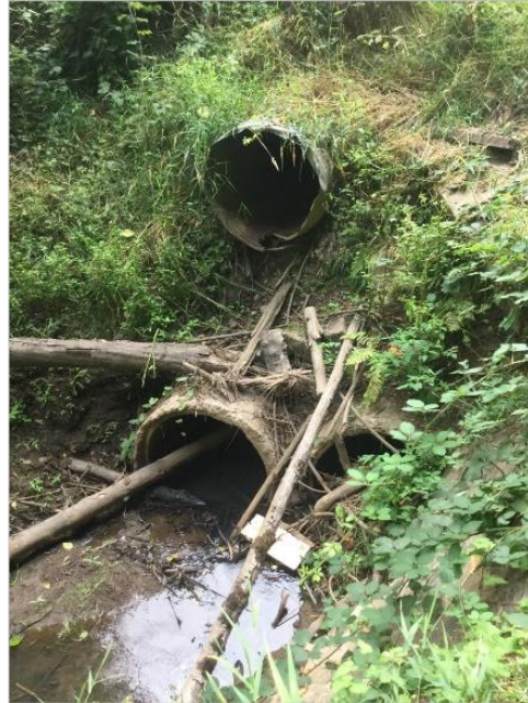
Photo 28. Culverts on east side of corridor, looking east.
