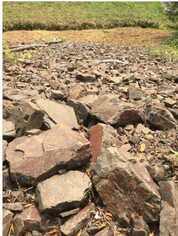
Photo 53. Riprap on slope on east side of rail berm, looking east and down.
