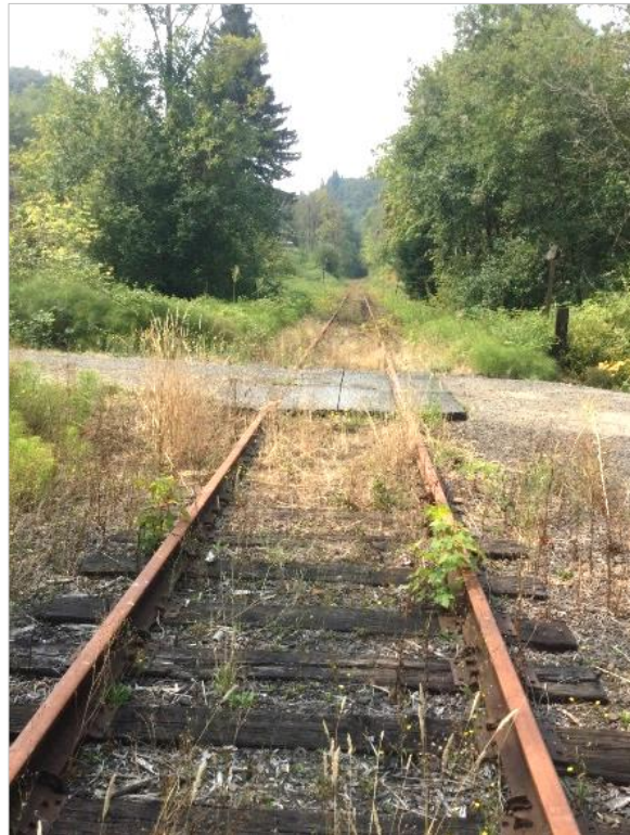
Photo 49. At-grade crossing on Evergreen Spur Road, looking south.
