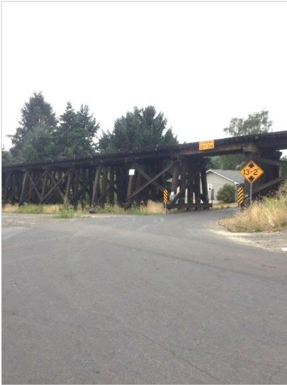
Photo 31. Trestle at Beulah Drive, looking southwest.
