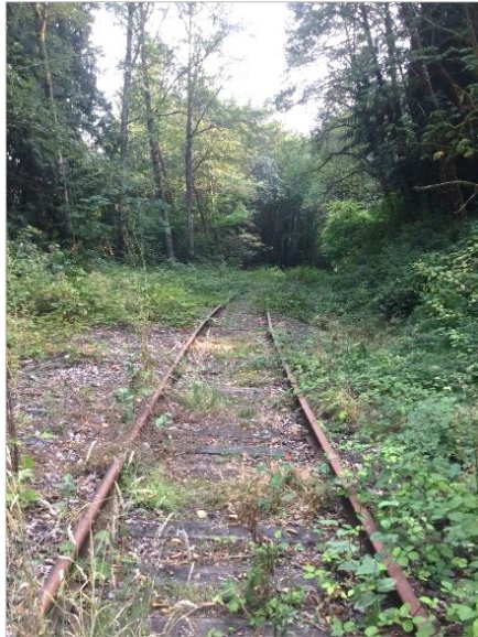
Photo 60. Corridor heading to Ostrander Road through a shaded area, looking north.
