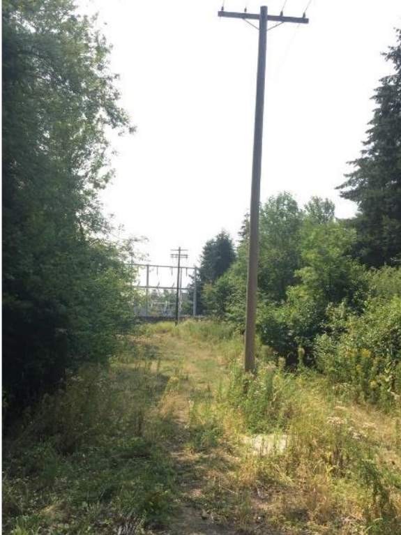
Photo 17. Electric utility and substation, looking south
