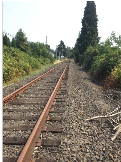
Photo 11. Rail corridor, looking east.
