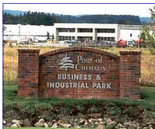
Port of Chehalis received an EDA grant to complete the first phase of the Port's Incubator Facility that will focus on energy in conjunction with the Centralia College Center of Excellence for Energy
