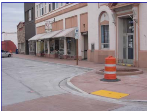
City of Castle Rock is completing a multi-phase infrastructure project throughout its downtown
